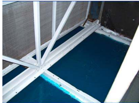
Typical Completed Pancrete Application for Pans & Horizontal Supports
